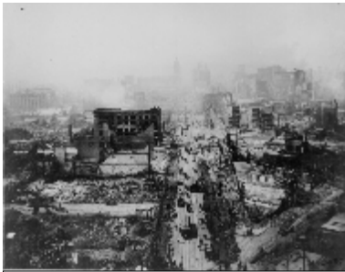
San Francisco earthquake 1906
