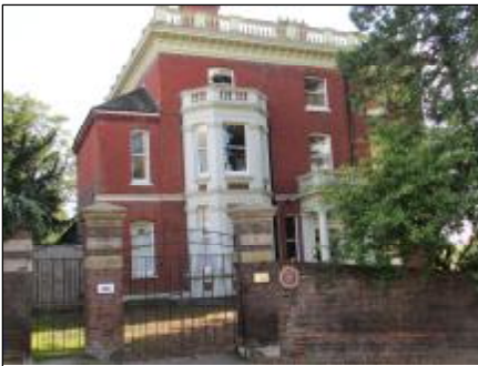
Torrington House, St Albans (2015)
